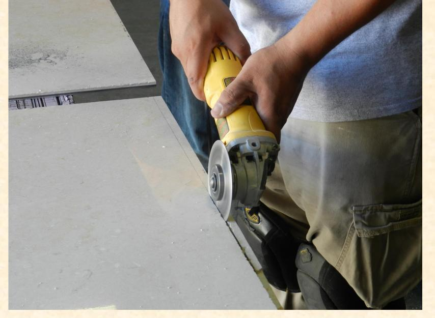
• When making irregular cuts, we suggest a 4 1/2" variable speed grinder with an unsegmented diamond tip blade.
