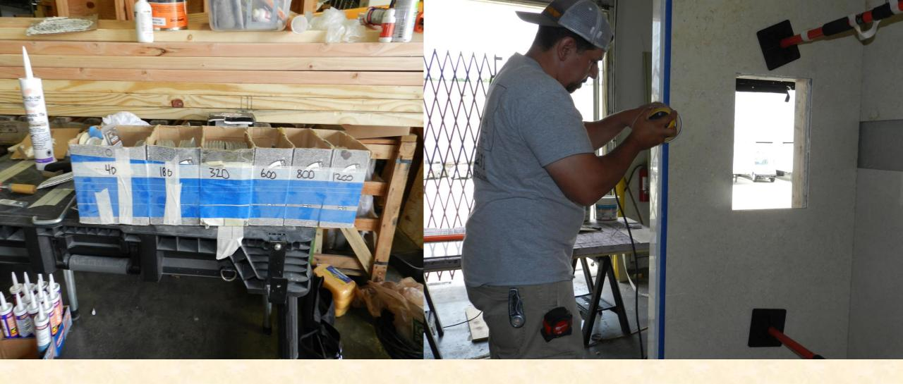
To ease and polish the mitered edge, <u>use very high grit paper</u> with an orbital sander. Higher grit paper is used for marble (600-1200).
