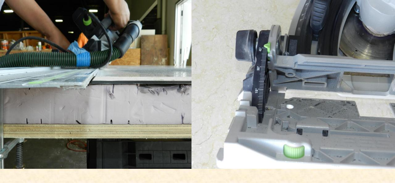
To make the wrap around effect, 45 degree miter cuts are used. Angle the blade to cut at 45 degrees and cut using the track, go steadily and carefully. The stone is then dry fit to check your cuts before gluing.
