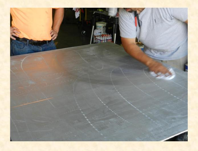
• To attach stone to the walls, we use a combination of adhesives. We used Latapoxy 310 2 part adhesive and Loctite PL 375 Heavy Duty adhesive; silicone can be added as well (many other adhesives can be used). Clean the aluminum side off before installing.
