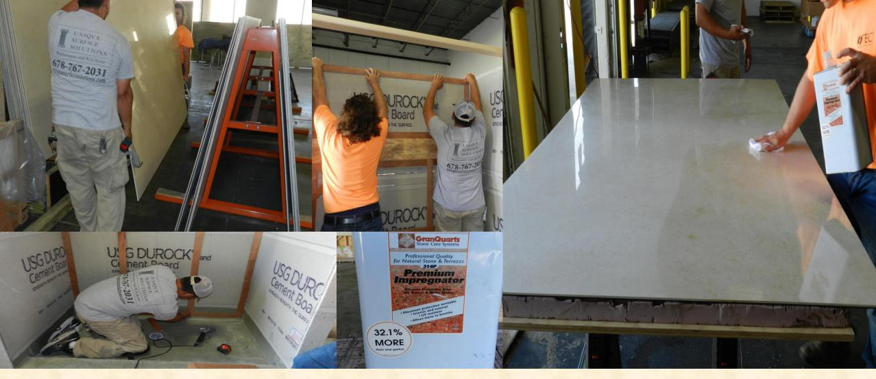
First, be supervised by an experienced ThinSlabz™ installer to properly handle material. The sub-wall you work with needs to be suitable for setting stone. Waterproof all areas as you would for normal stone installations (when applicable). You will need to be working with a <u>clean</u> and <u>sealed</u> slabz.
